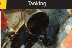
Tank the recess with hot BJ200 binder to seal the joint and improve adhesion of the joint to the asphalt.
