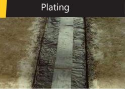
Install the aluminum strip or steel plate over the gap Materials (the steel plate size according to fig.1).
