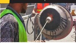
a-The aggregate must be heated in a vented rotating drum mixer by the use of a hot compressed air lance. The aggregate has to be heated to a temperature of 150°- 190° C.
