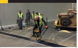
Compaction should take place as soon as possible after filling using a vibratory plate or roller.
