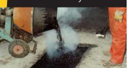
The hot pre-mix prepared shall be transferred to the joint and spread to a slight overfill in to layers.
